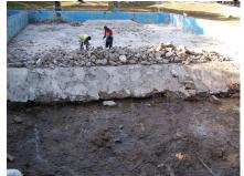
pool, due to major problems, cracks, and leakage of water.
