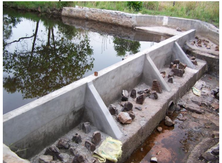
Front view of the dam, (raised 8 inches.).
